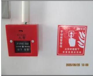
Photo of fire safety equipment Fire alarm.JPG
