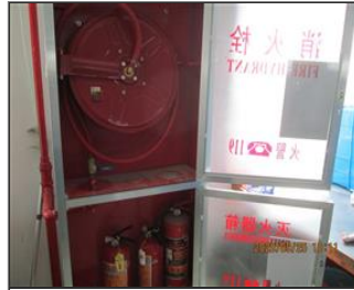
Photo of fire safety equipment Fire equipment.JPG
