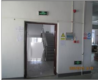
Photo of fire safety equipment Emergency exit.JPG
